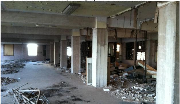
Photo 10 of 19 Photograph showing the terrazzo flooring still located on the first floor of the addition and the hallways on floors two through six of the original structure.
