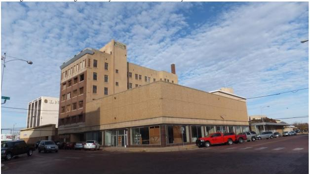
Photo 2 of 19 Looking northeast at the original cornice and detailing of the sixth floor, partially covered by metal paneling.
