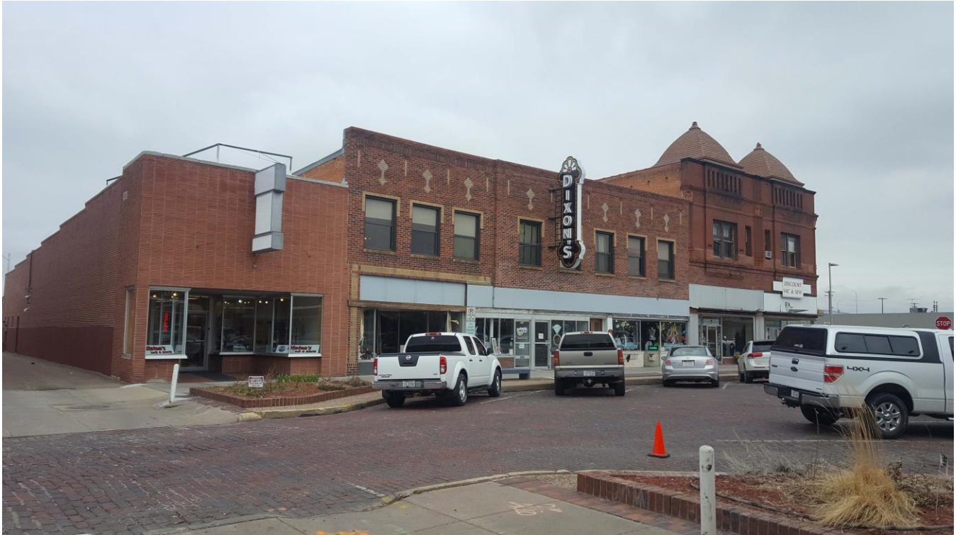
6. The west side of the 500 block north of the alley on Dewey Street.
