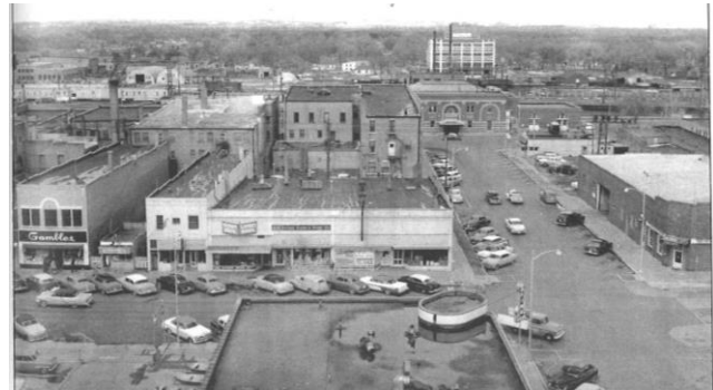
Figure 11: North Bailey Street, looking North towards Union Pacific Depot; All the buildings have been demolished (Source: North Platte: City Between Two Rivers)
