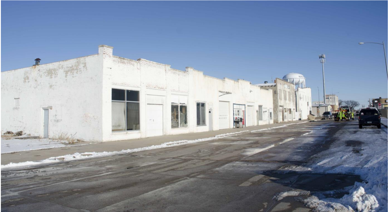
26. View of West 7 th Street looking east from the intersection of Vine Street.
