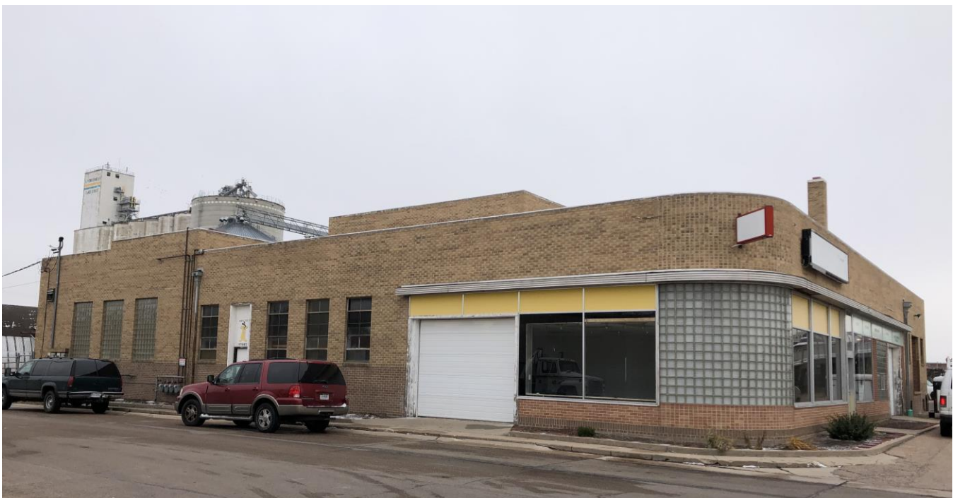
27. View looking south from the intersection of North Jeffers Street and East 7 th Street.
