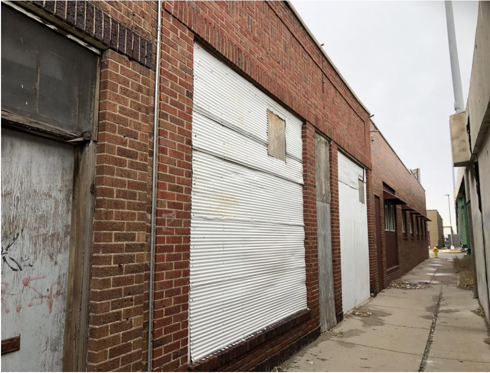
20. View looking north adjacent to the west side of the Jeffers Street viaduct.
