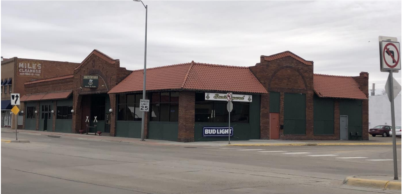
18. View of the Firestone Garage looking southwest from Jeffers Street and 6 th Street.
